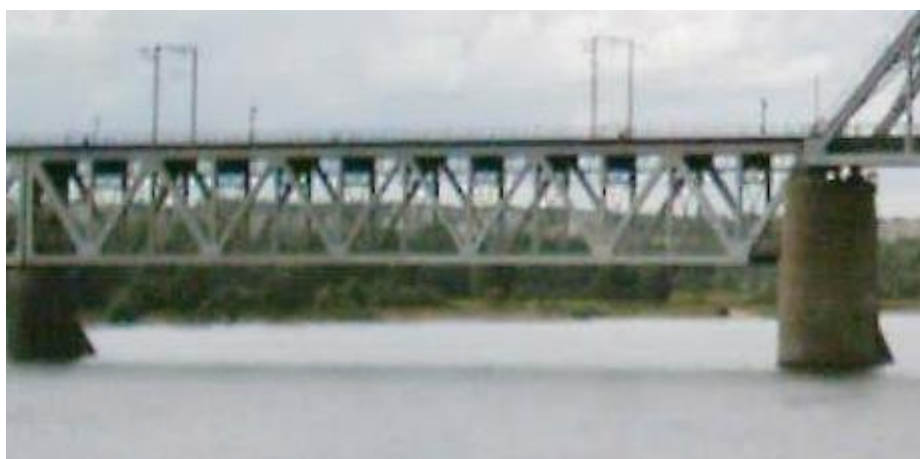
Figure 2 — one of the bridge spans
